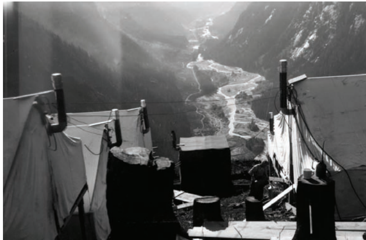
LEFT: WORKERS INSTALLING ALCAN POWER LINES LIVED IN TENTS IN KEMANO
